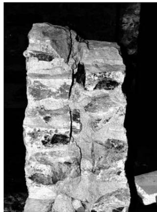
Figure 1.1: Double-leaf masonry (wall cross section)
