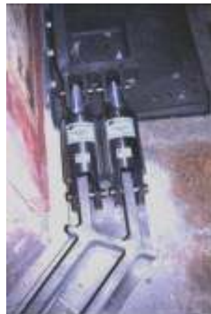
Figure 3.10. Particular of the SMA device utilized for the seismic upgrading of the Basilica of St Francis in Assisi, Italy.
